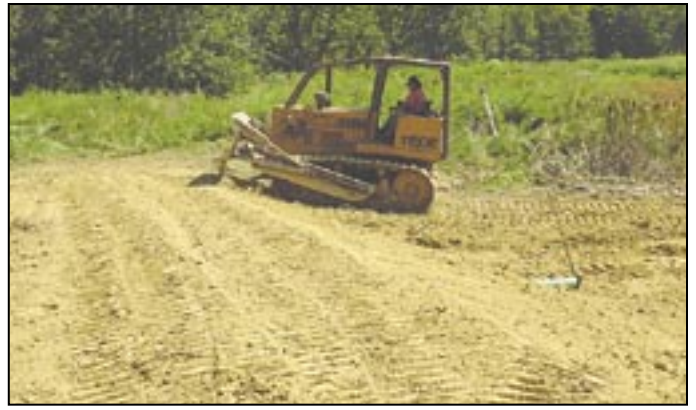
Pack the dam in layers.
