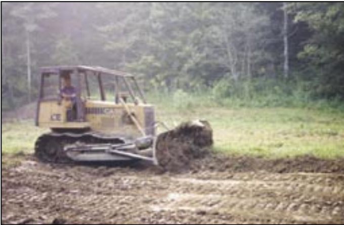
Remove and save topsoil.
