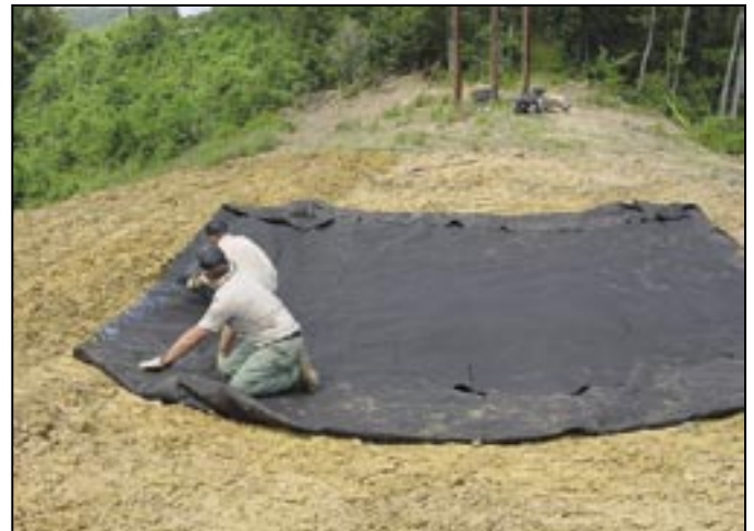
A liner is placed in the depression.
