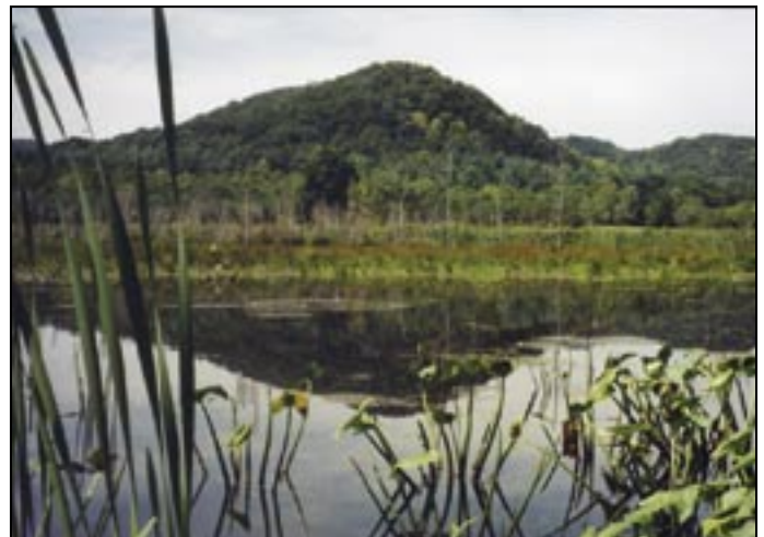
Five-year-old wetland built with a track-hoe and dozer.
