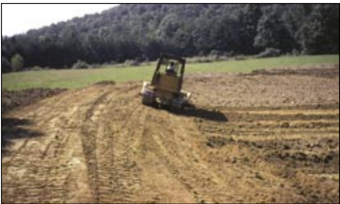
Make gradual slopes on the dam.
