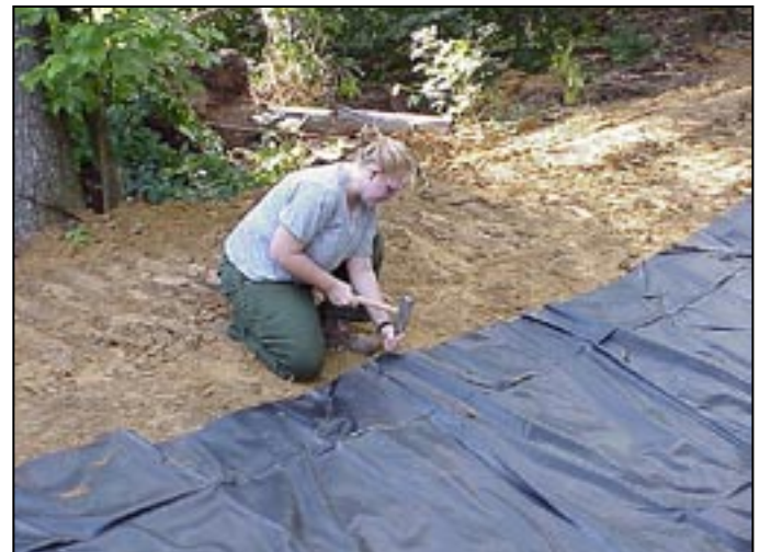
The liner is secured with stakes.
