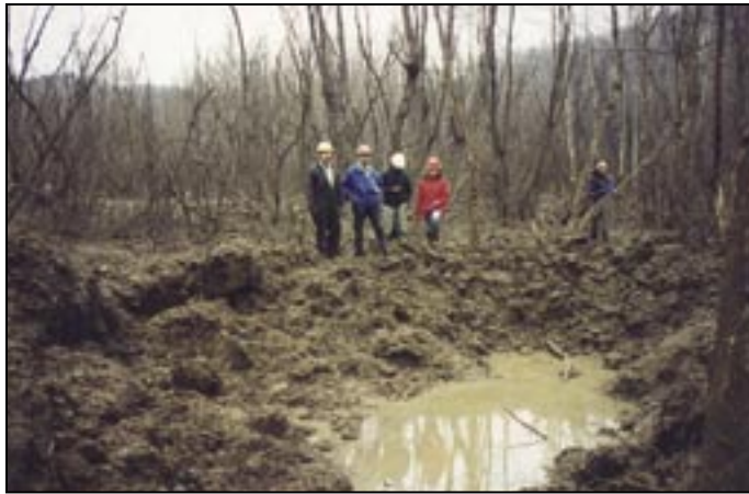
Site immediately after blasting.
