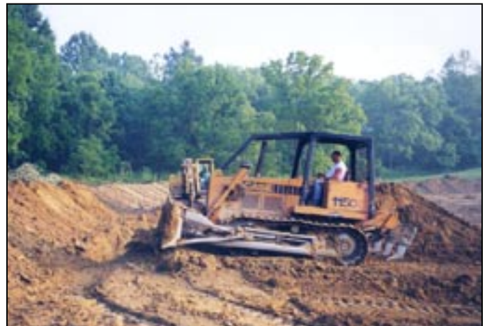
Dozer packs soil in layers to build a dam above the core.
