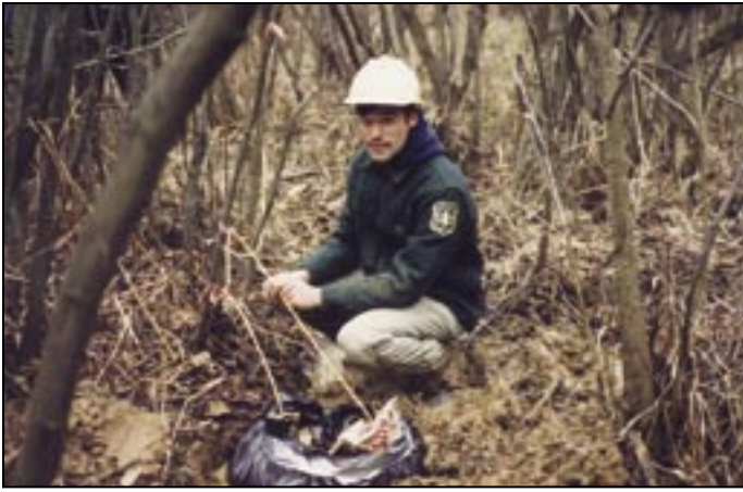
AN/FO is placed in a shallow hole.
