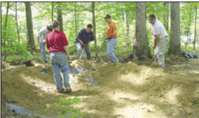
After placing the liner, they covered it with soil.
