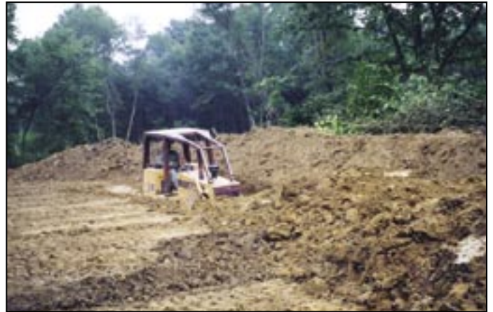
Make a core under the dam location.
